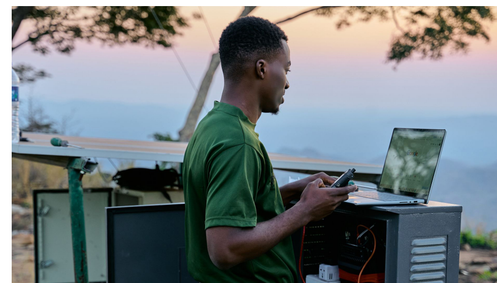
CCT Technology Officer Simbai Mutematembi on Chirambakudoma Mountain during installation of the new digital radio communication system
