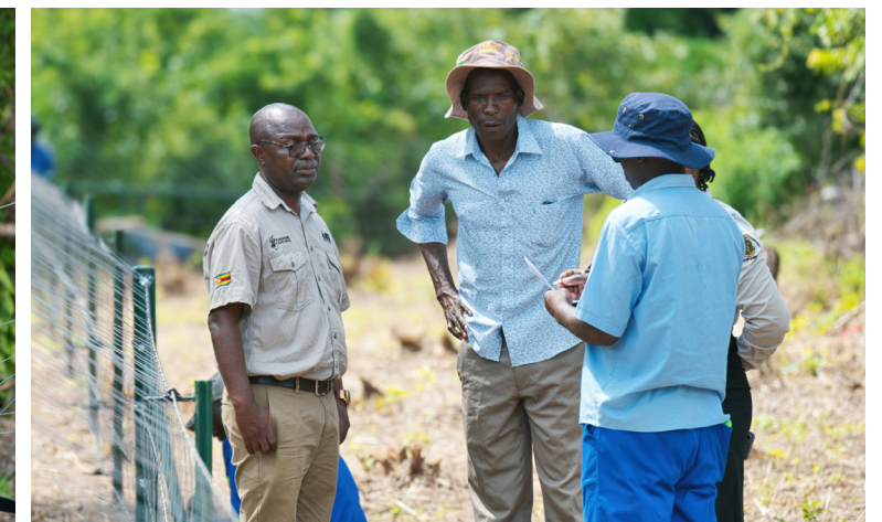
CCT Community Manager Simba Sandram discusses fence installation progress with the lead fence installer and Promotion Dzomba, Masoka Ward Secretary
